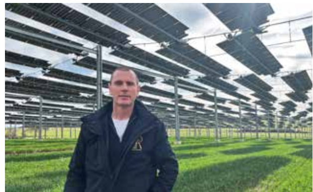
Sylvain Raison is taking part in the photovoltaic roof project in the Haute-Saône department.
